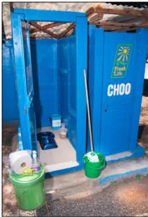
In Kenya, Sanergy's "Fresh Life" toilets use a urine-diverting squat plate
