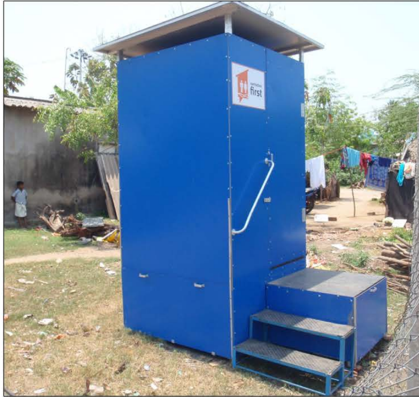
Metal frame, walls and roof. Photo: Sanitation First
