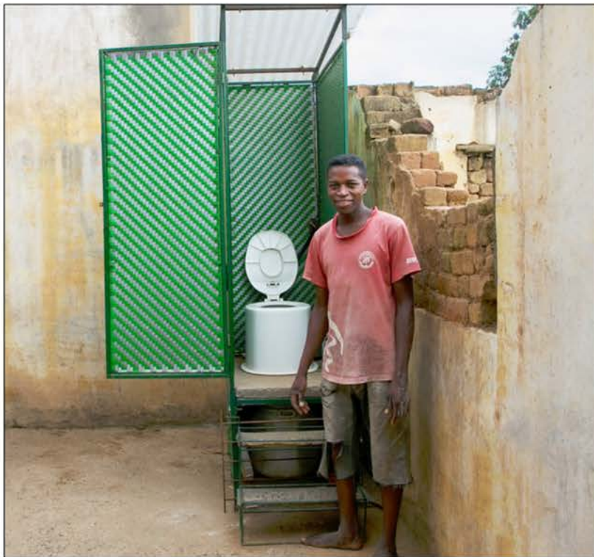
Metal frame with woven plastic walls. Photo: Loowat
