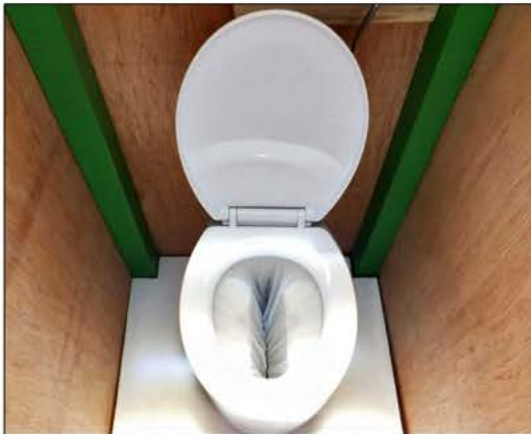
In Madagascar, Loowatt provides waterless-flush sanitation systems that seals waste into a portable cartridge using biodegradable film, which prevents odors and does not require any cover material
